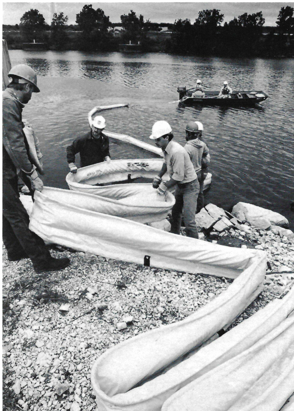
Practice makes perfect, the old saying goes, and participants in North Line's boom deployment exercise put this theory into action. Working together, Pipe Line employees and others deploy a boom across the waterway at Argo facility's docks.
